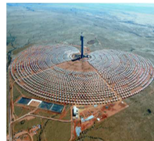
Khi Solar One 50 MW Tower with energy storage system
