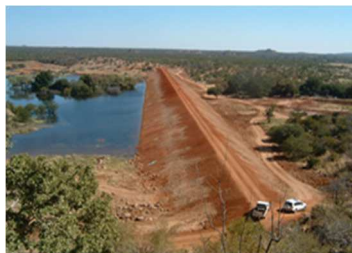
Construction of Border Dam: Gravel Embankment Dam: Dam Engineering Services
